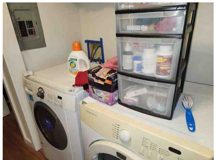
Laundry and Electric Unit B
